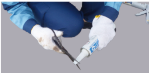
2. Cut the nozzle at the appropriate position
