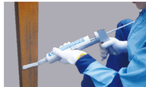
5. Apply LEAKMASTER LV-Z continuously without a break to the place to be sealed
