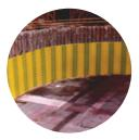
Curved or complicated foundation forms can easily be produced on-site.
